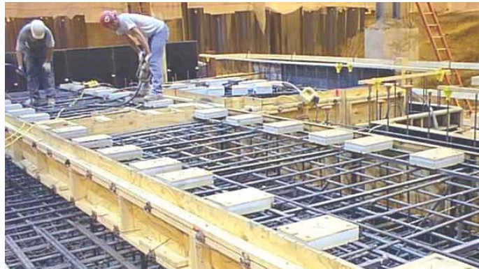
Caterpillar C175 Machine Foundation
